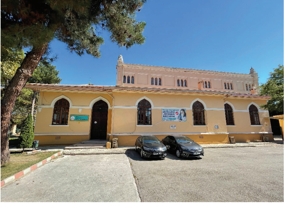
G. 6: Edirne Union and Progress Club Building, West Front View, (A. Balci, 2022)
