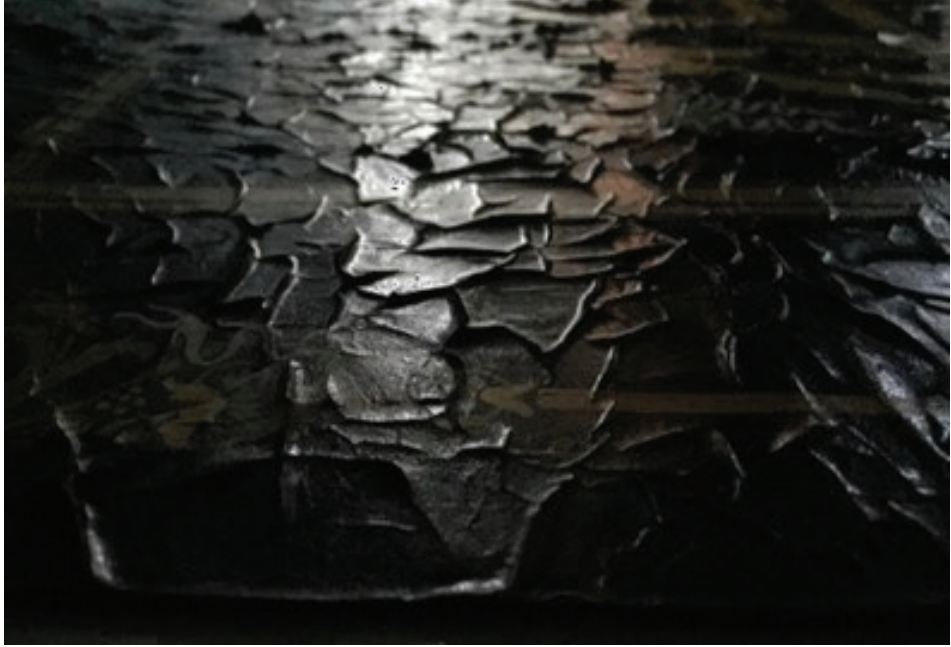
F. 17: Details in visible light (VIS)- Cracks and blisters parts of the paint layer (Gülder Emre, 2019)
