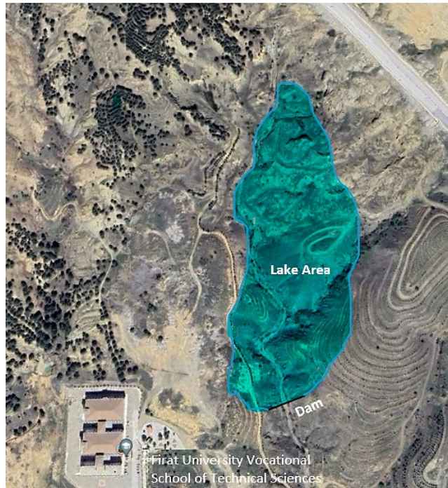
Figure 1. General view of the project site.
