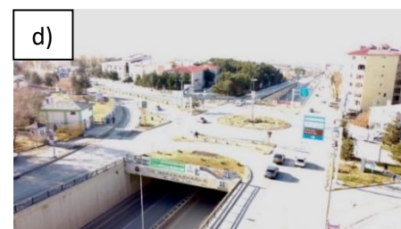
d. Central Median Visibility (Gürbüz, 2021)
