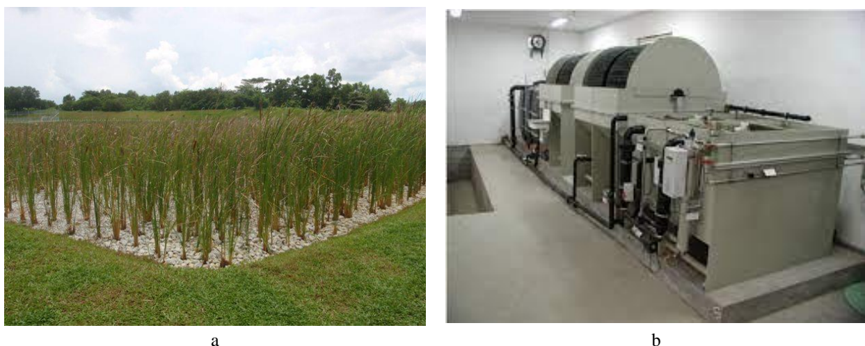
Figure 1. Greywater treatment technologies: a) Constructed wetland [21], b) Rotary biological reactors [12], c) Sequential batch reactors [22], and d) Membrane bioreactors [23]
