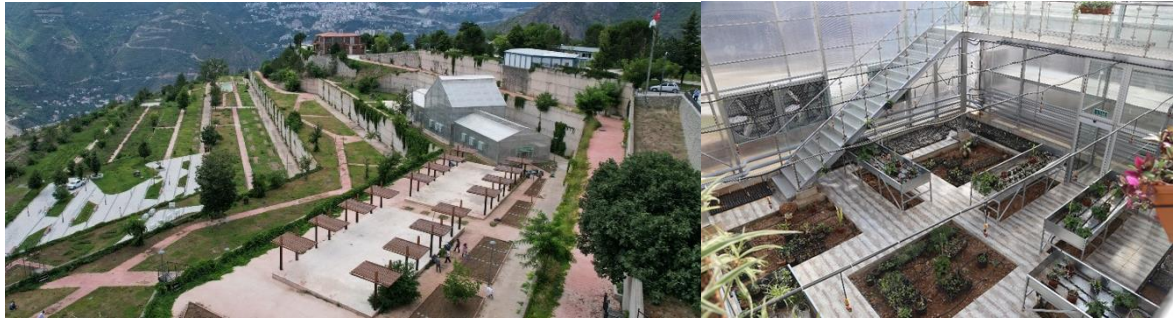
Figure 7. General view of the R&D and Exhibition Greenhouse
