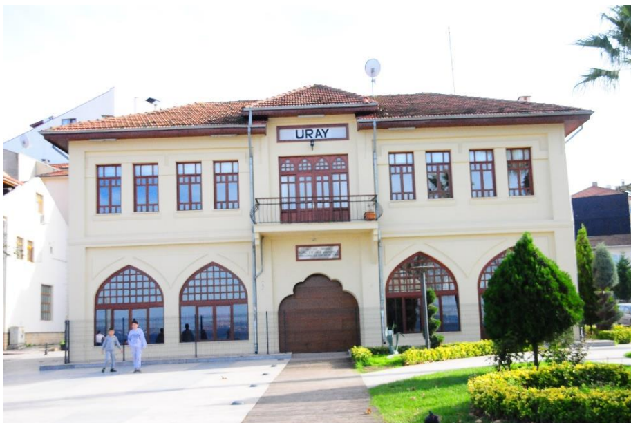
Figure 13. Entrance Facade - Northwest Façade
