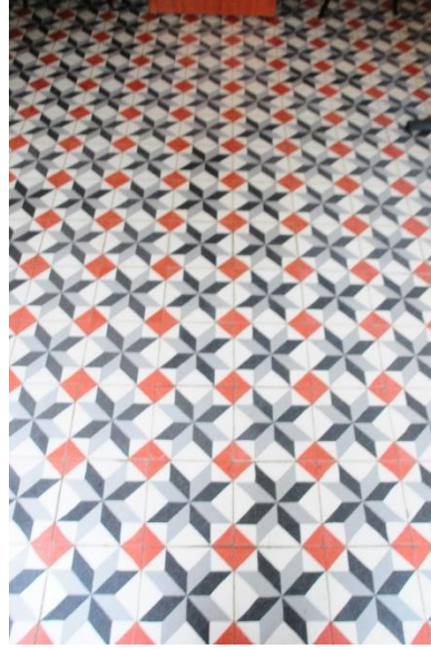
Figure 18. Ground Floor Tile Coating
