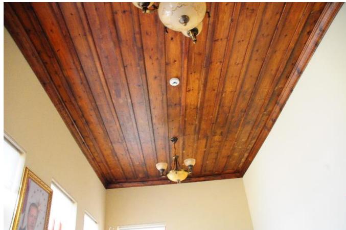
Figure 17. Interior Ceiling Coating
