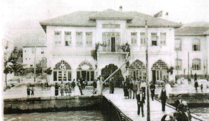
Figure 12. An Old View of Karamürsel Municipality Building [Karamürsel Municipality Archive] [26]
