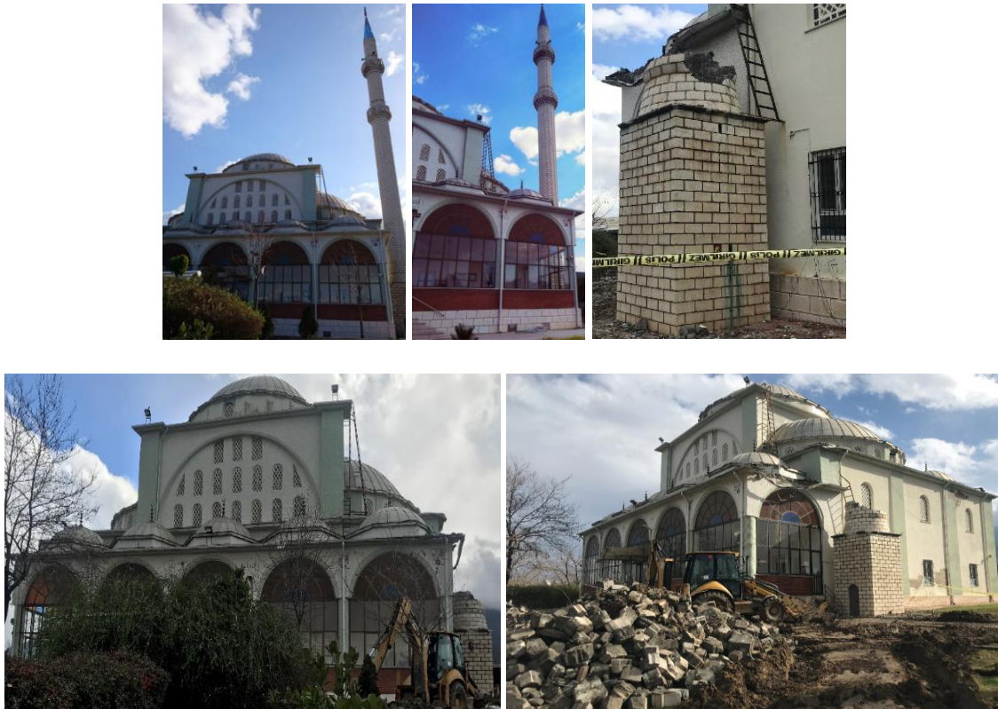
Figure 3. Before and after the collapse of the minaret of Industry Mosque
