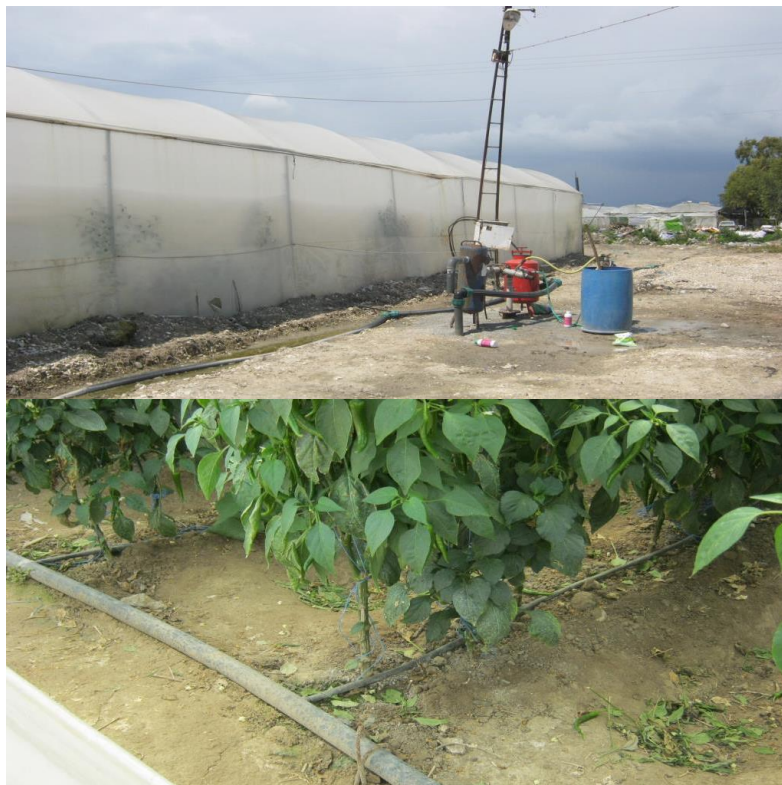
Figure 4. Water supply, drip irrigation system and control unit in greenhouse
