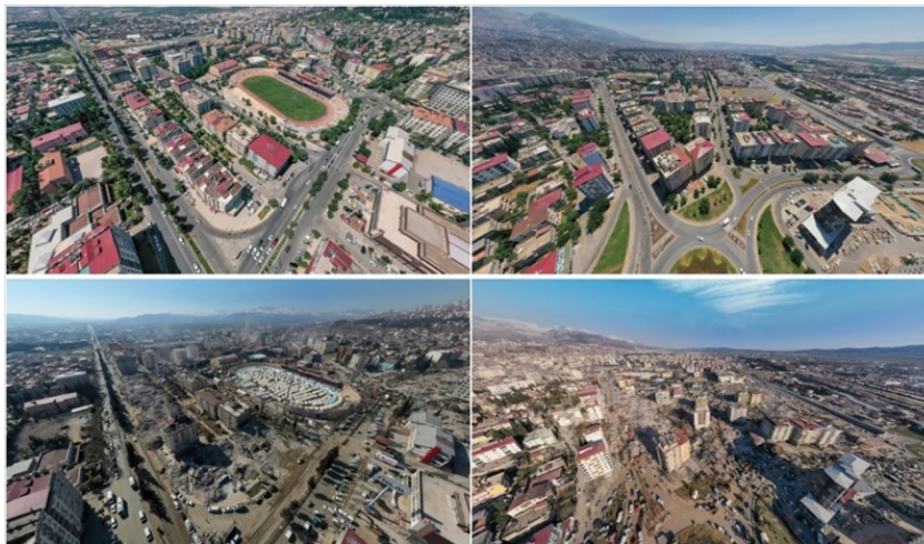
Figure 1. A view of Kahramanmaraş before and after the earthquake (Kara, 2023)
