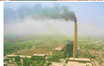
Figure 1: The Dora power station, on the right: an aerial photograph from Wikimapia and on the left a screenshot from GoogleEarth.
