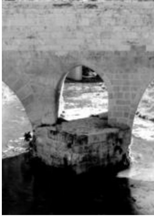
Figure 5. Discharging Arch in the West (Photo: İ. Göçmen)
