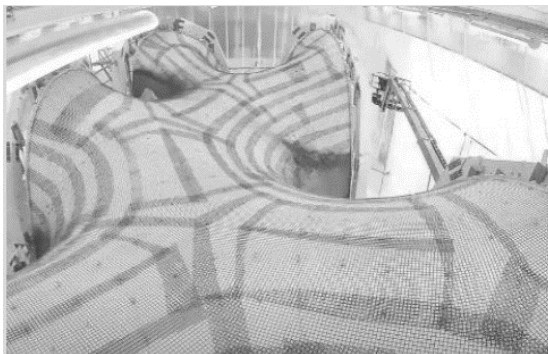
Figure 9. Images of Hilo Shell structure (ETH Zurich., n.d.). Full-scale construction prototype: NEST HiLo shell roof) (Mele et al., 2017).
