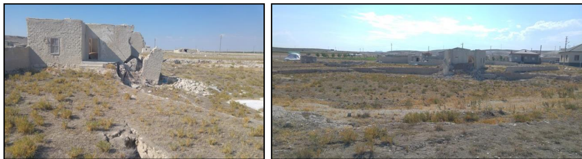
(h) A new sinkhole formed within the settlement in 2014 (Diameter: 50 m)
