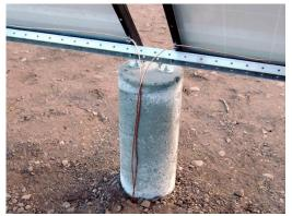
Fig. 13. Grounding for a solar PV system [32].
