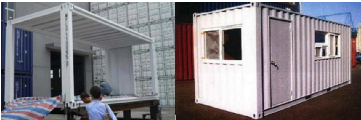
Figure 8: Left: Plus Box Frames Right: ISO converted frame, (Hikone & , Tokubuchi, 2011)
