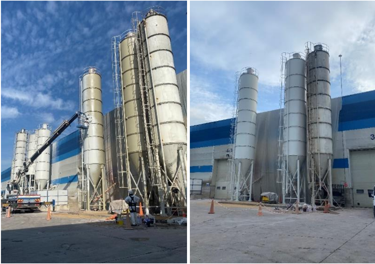
Figure 12. Topcoat paint application of silos
