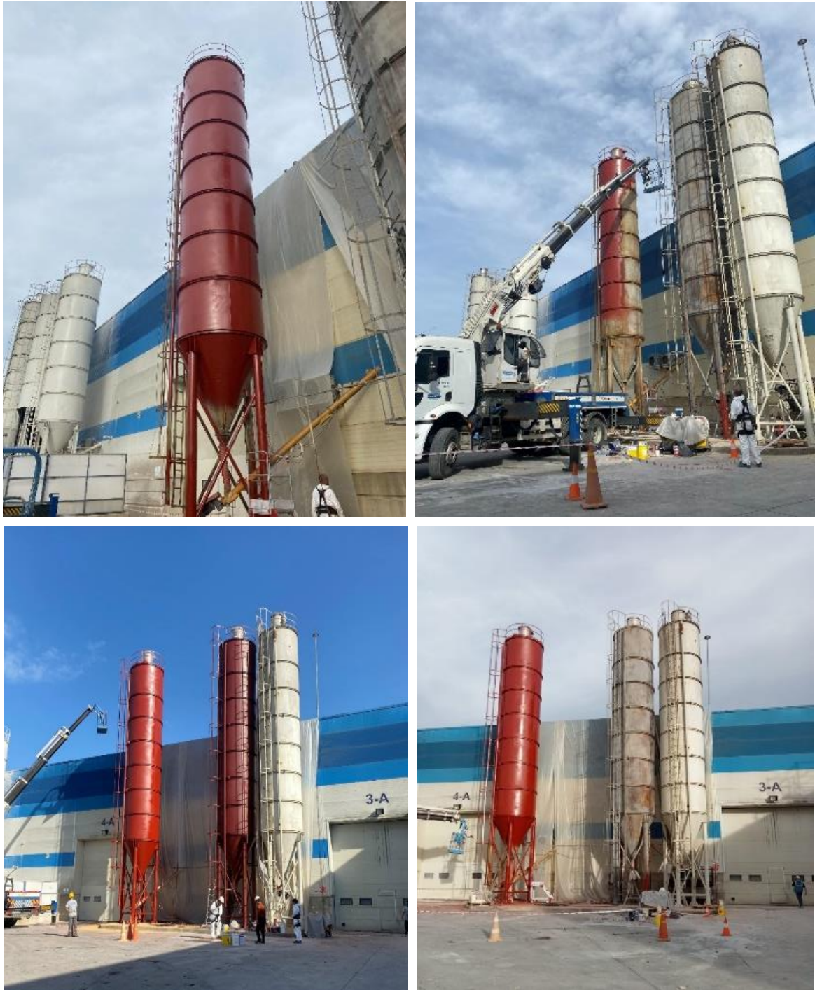
Figure 9. First coat primer application
