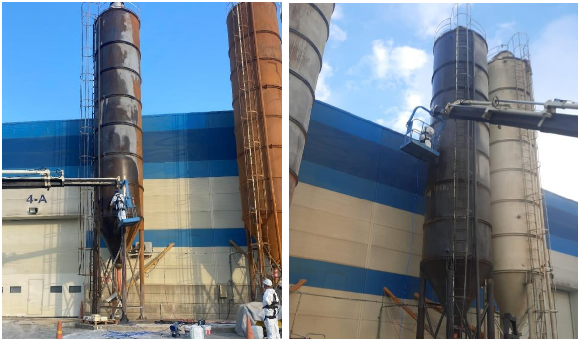
Figure 6. Washing process with chemical solution
