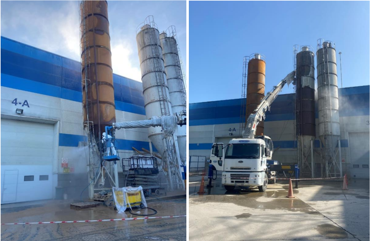
Figure 4. Wet blasting process
