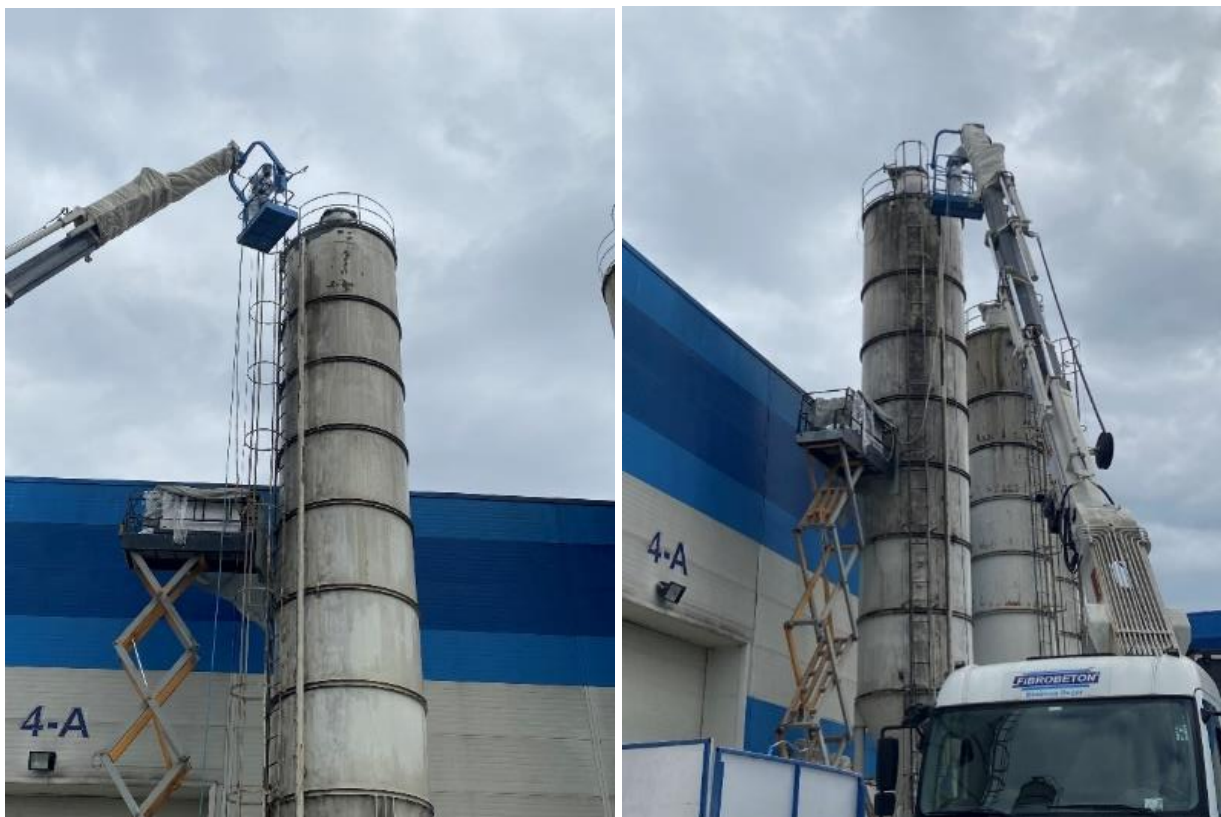
Figure 2. First state of silos
