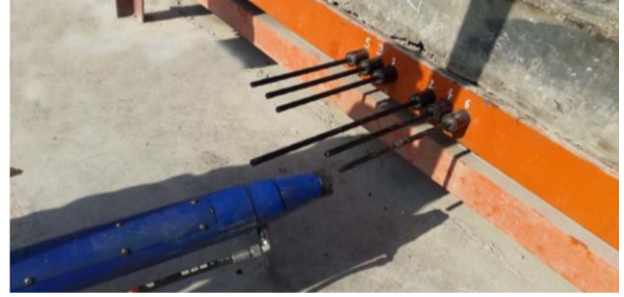
Figure 13. Pre-tensioning application
