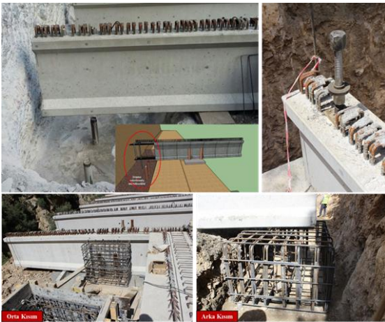
Figure 10. Estacade beam and bolted connection placed to be connected to micro piles
