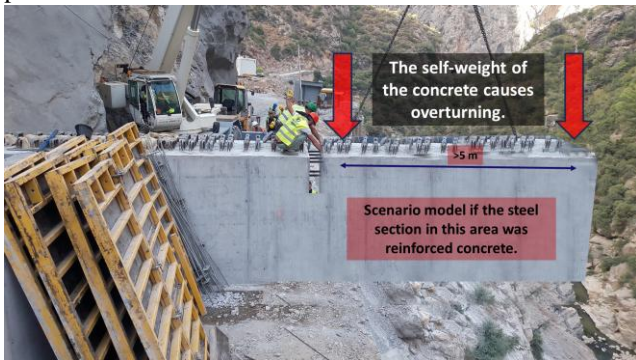
Figure 16. Assuming that the Type-3 beam is entirely reinforced concrete
