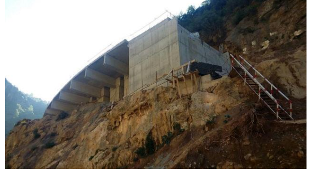
Figure 17. Bottom view of the road built with the Estacade system
