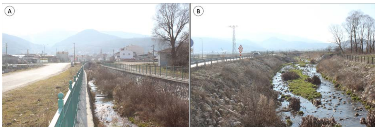
Figure 3: The channel structure in different parts of the Değirmen Stream, which passes through the district center.
