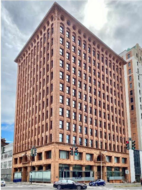
Figure 3. Louis Sullivan and Dankmar Adler's Guaranty Building (Prudential Building), built in Buffalo, New York in 1896. (URL-5)
