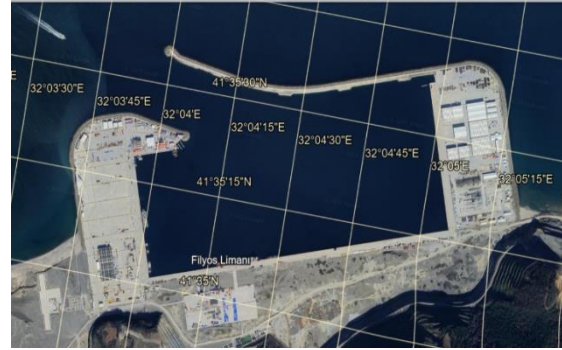
Fig. 2. Satellite View of Filyos Port (Google Earth, 2024).
