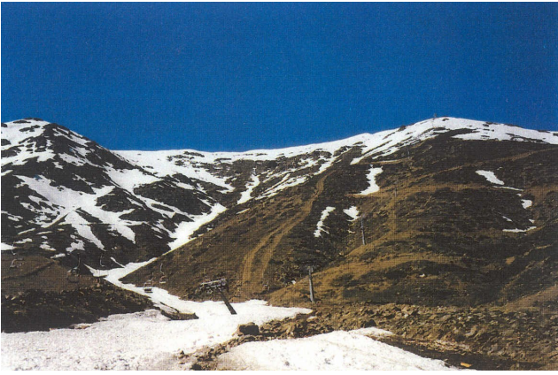
Figure 4. Condition of Skilift Poles After Avalanche Incident in Bozdağ (2015)
