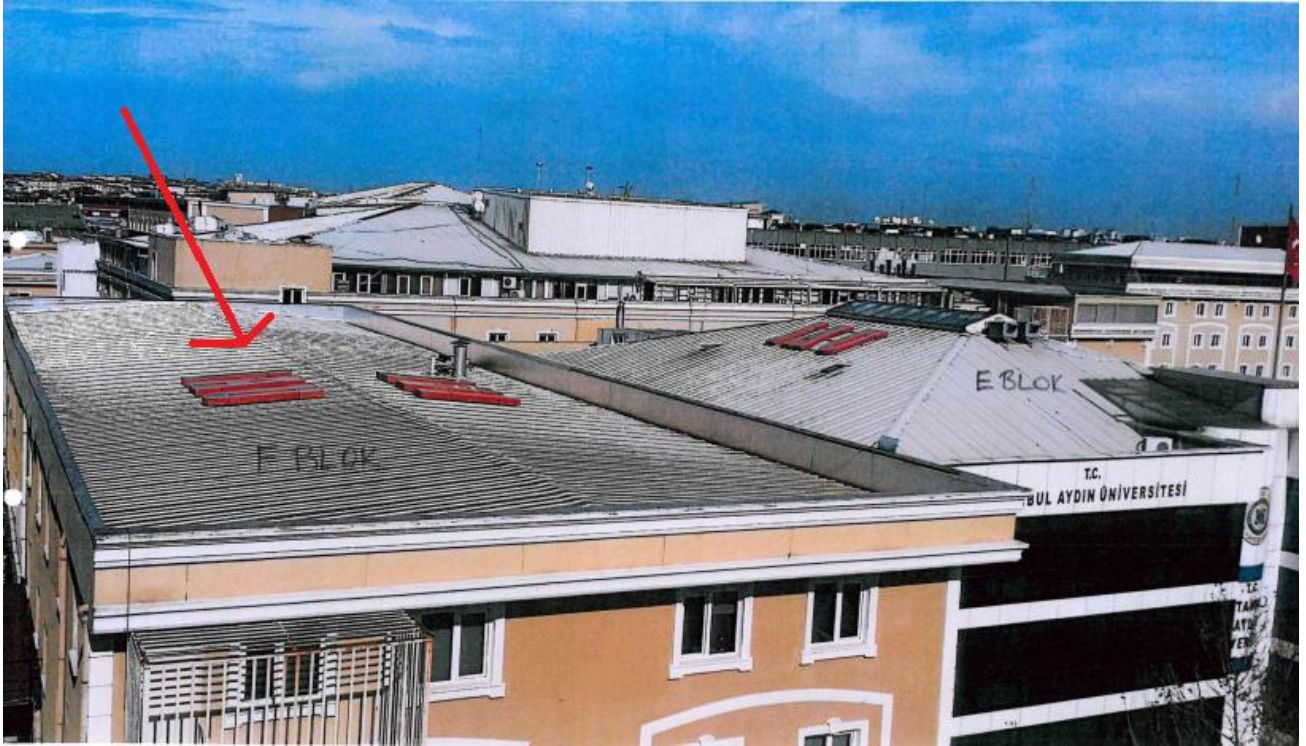
Figure 3. Rooftop of block F
