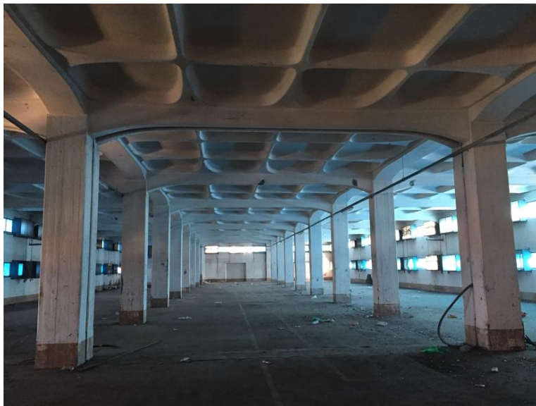
Figure 37. Concrete slabs of the tobacco factory, 1949-1933, Bologna (Antonucci & Nannini, 2019).
