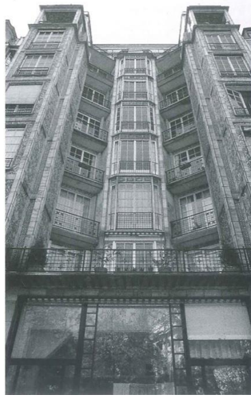
Figure 33. Facade of the Franklin Apartment, Paris, France (Moffett, Fazio, & Wodehouse, 2004).
