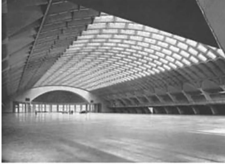
Figure 36. P.L. Nervi, Central hall (Hall B) of Turin Exhibition Complex, Turin, 1948 (Chiorino & Chiorino, 2011).
