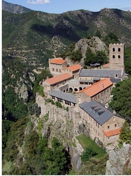
Figure 13. View of the Monastery of Saint Martin (Janberg, 2022).
