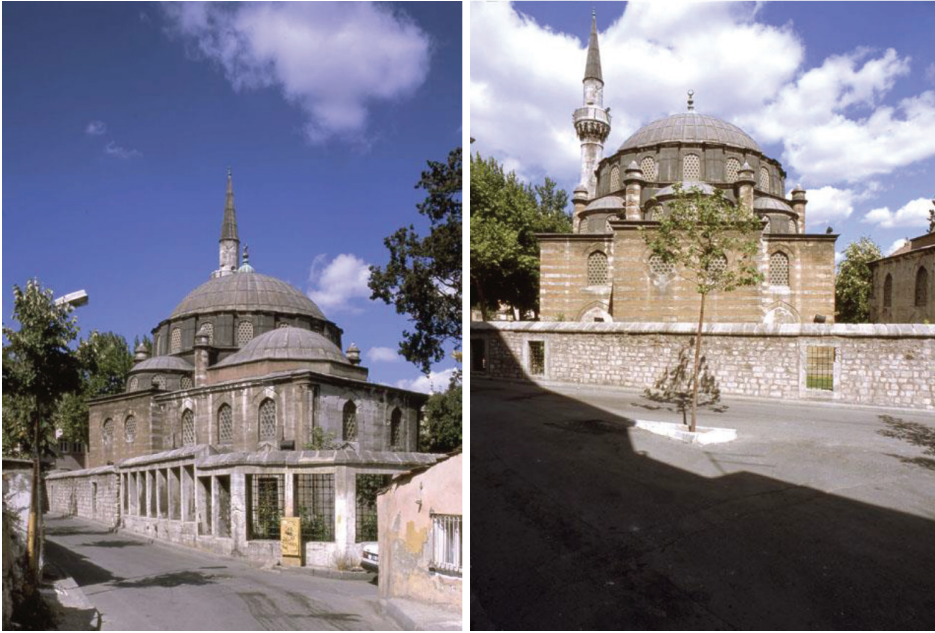
Fig. 4 Habeşi (Abyssinian) Mehmed Agha complex in Çarşamba neighborhood, in Fatih district (Photographed by Reha Günay, courtesy of Gülru Necipoğlu, The Age of Sinan: Architectural Culture in the Ottoman Empire , (Princeton and Oxford: Princeton University Press, 2005, Fig. 524 and 525, p. 499)
