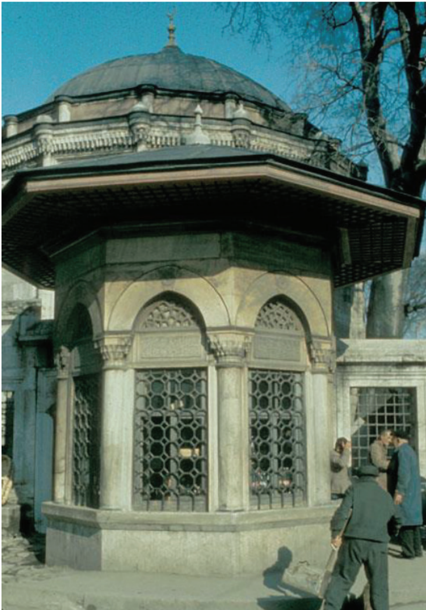
Fig. 17 View from Yeniçeriler Street, looking east towards sabil and tomb Koca Sinan Pasha Complex (Photographed by Walter B. Denny, courtesy Aga Khan Visual Archive, MIT)
