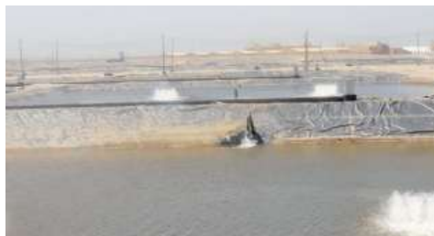
Figure 4. Construction Works at Birkat Ghalioun Project. (Photo Credit: Al-Ahram Daily, Egypt)
