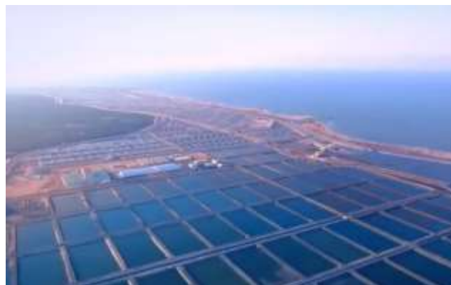
Figure 5. Construction Works at Birkat Ghalioun Project. (Photo Credit: Al-Ahram Daily, Egypt)
