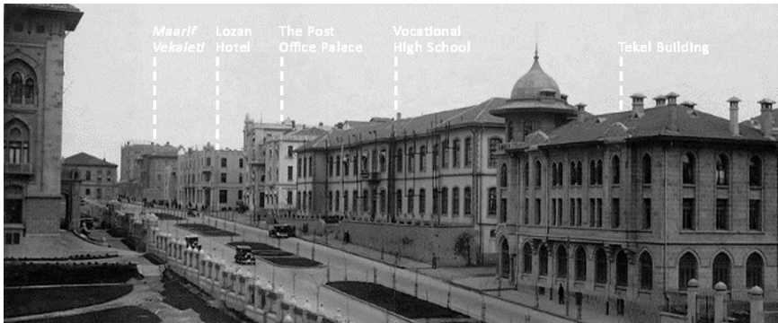
Figure 11. A postcard showing the east side of Atatürk Boulevard, going towards the Post Office Palace. (Archive of fotoankara. Adapted by the author).
