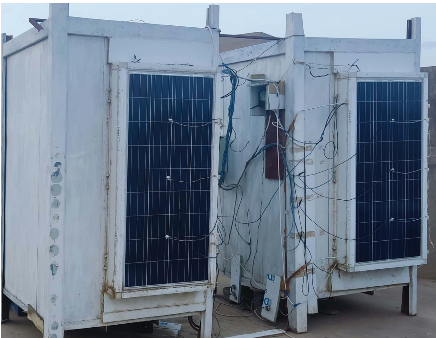
Figure 2. The exterior appearance of the PV/Trombe wall.
