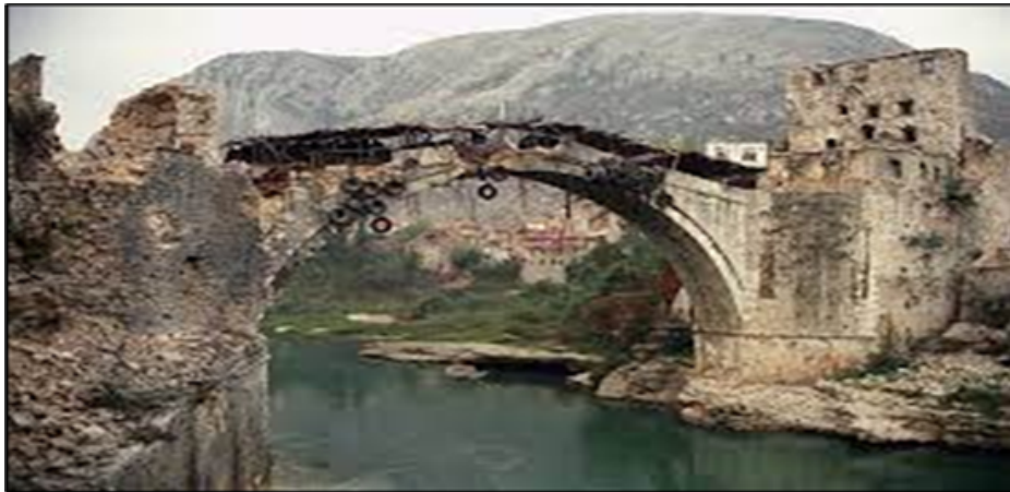
Demolished Mostar Bridge
