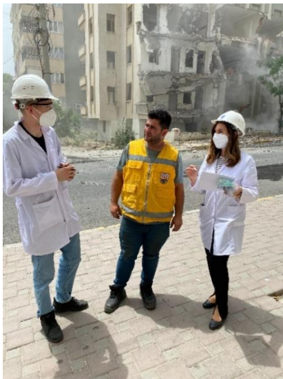
Figure 4. Conducting a survey in the severely damaged building demolition area.
