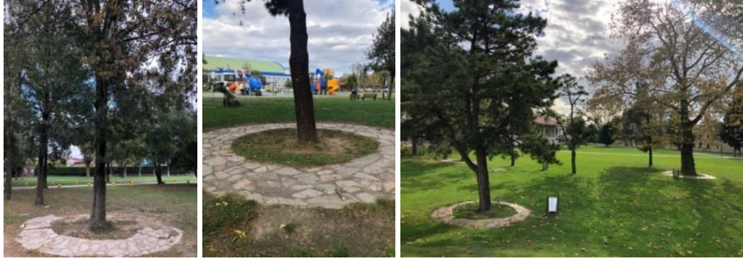
Figure 24. Photographs from the stone paving application at the base of trees (Authors)
