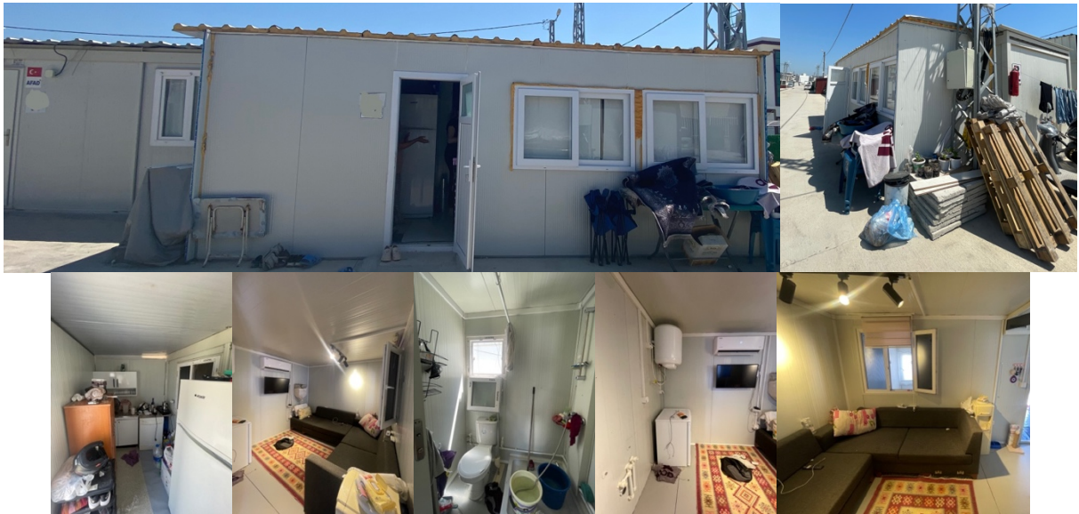
Figure 5. Examples of personalization in the facade and interior of the container (Tarakçı, 2024)
