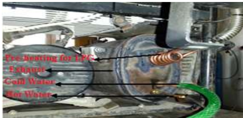
Figure 2. Water connection to the heat exchanger and preheating of the LPG on the exhaust
