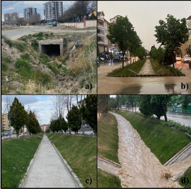
Figure 3. Culvert inlet (a), outlet (b) and open channel downstream of the culvert (c, d)
