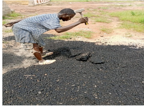
Figure 2. RAP in Manual Crushed State
