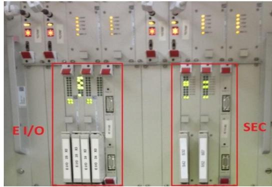
**Figure 3.** Electronic input/output and signal electronic control cards
