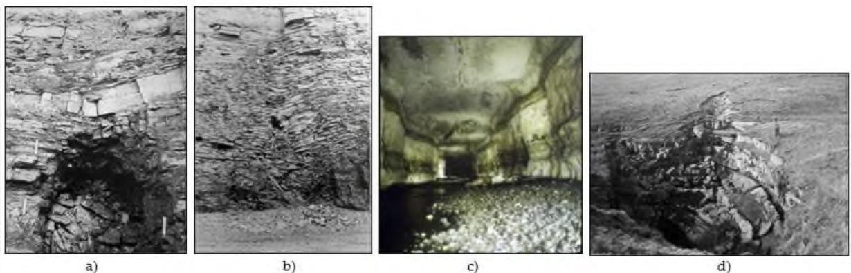
**Figure 1.** a) Roof collapse at an abandoned coal gallery inherited with thick overlying strata [2 & 3], b) Abandoned coal mine gallery which had been totally filled with caved overburden roof rocks [2 & 3]; c) Fracturing roof strata at Sof-Omar cave (Ethiopia), [4], d) Sinkhole formed at Yorkshire (England) due to collapse of roof layers at a limestone cave, [5].
