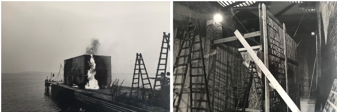
Figure 8. a. The burning of the container in the lagoon (ASAC, 1975: A.V.108.1975.8); b. Re-installing the container in the Magazzini del Sale (ASAC, 1975: A.V.108.1975.12b).
