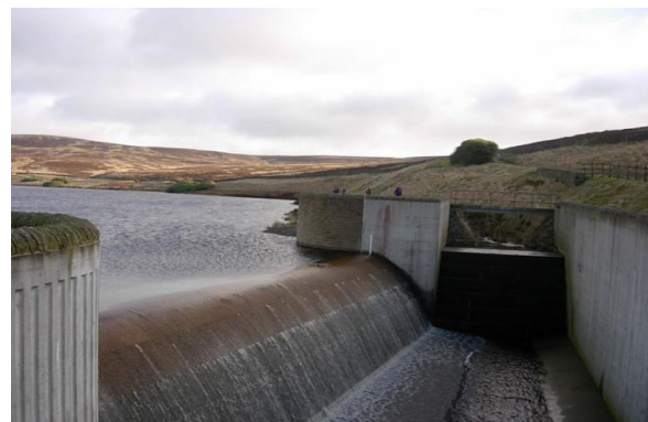
Figure 1. Walshaw Dean Reservoir [4]
