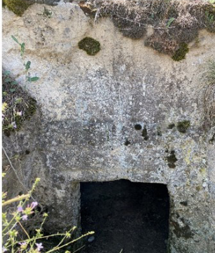
Gate facade with triangular pediment
