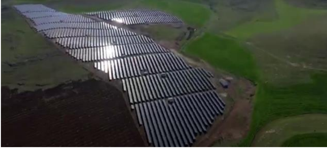
Figure 1. Images of the PV power plant.
