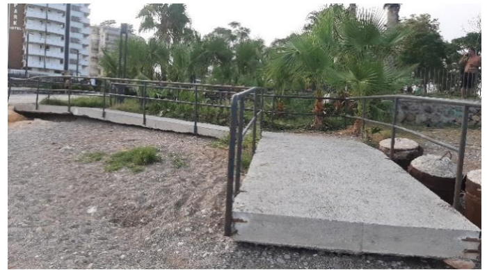
Figure 7. Ramp design is not suitable for accessibility (Çevrimli Archive, 2024)
