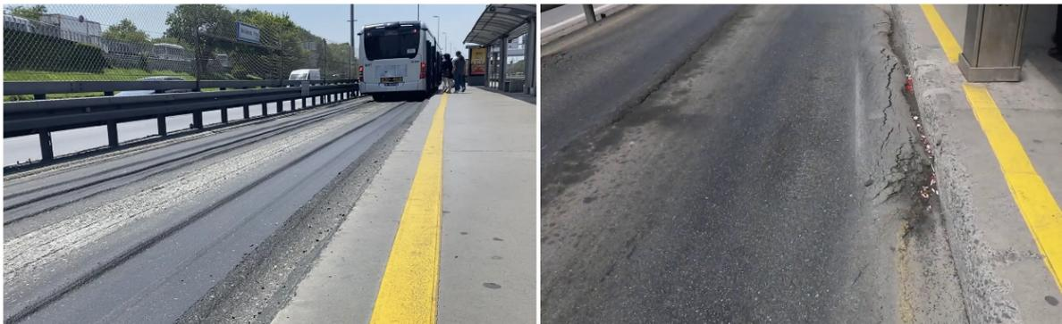
Fig. 1. Asphalt deterioration in Istanbul BRT line [31]
