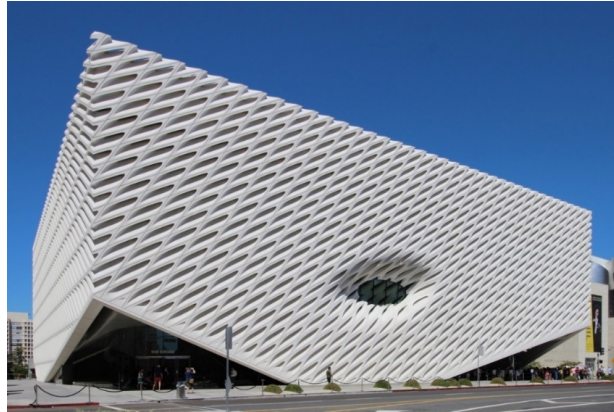
Figure 13. Broad Museum (Los Angeles, USA) (Material: GFRC-Glass Fibre Reinforced Concrete) by Diller Scofidio + Renfro ( www.wheristhenorth.com )
