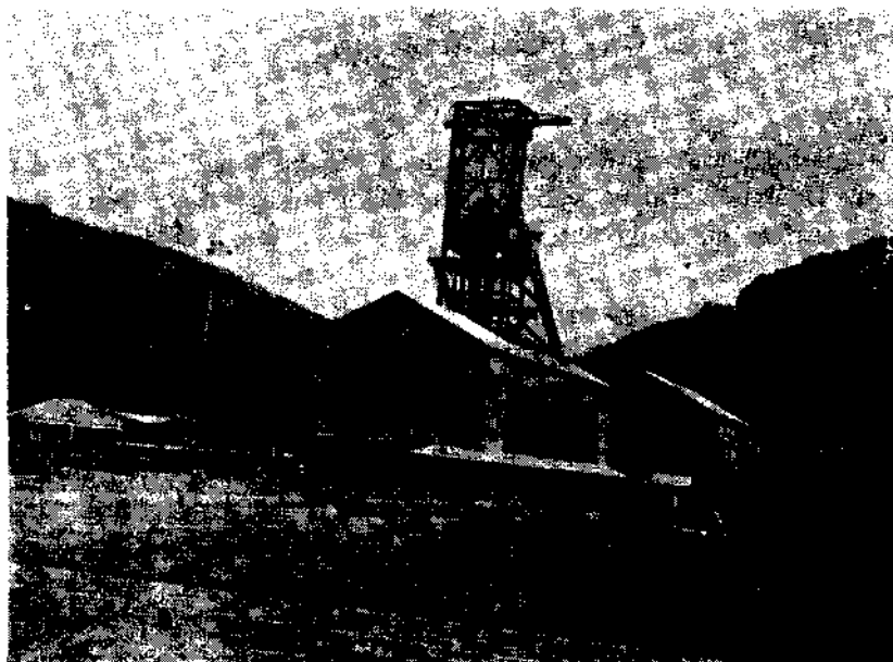
Fig. 4 - Shaft No. 1, Karadon district.
