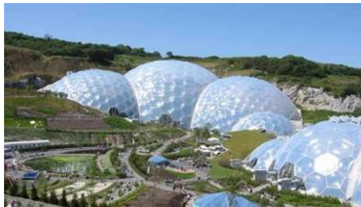
Figure 12. ETFE domes of the Eden project, UK [14].
