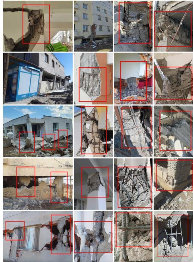
**Figure 4.** Examples of damage in columns caused by various factors (Photos taken by authors)
