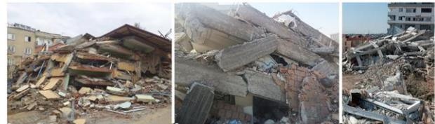
Figure 2. Examples of reinforced concrete buildings that have collapsed completely (Photos taken by authors)
