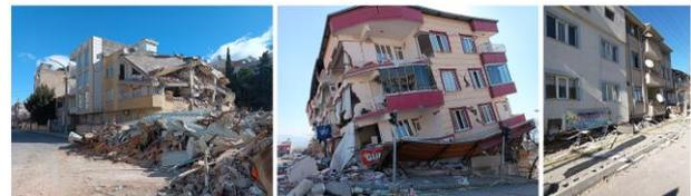
Figure 3. Examples of partial collapses due to various irregularities and deficiencies (Photos taken by authors).
