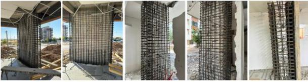
**Figure 9.** Example of the structural member strengthening with the jacking method (Photos taken by authors)
