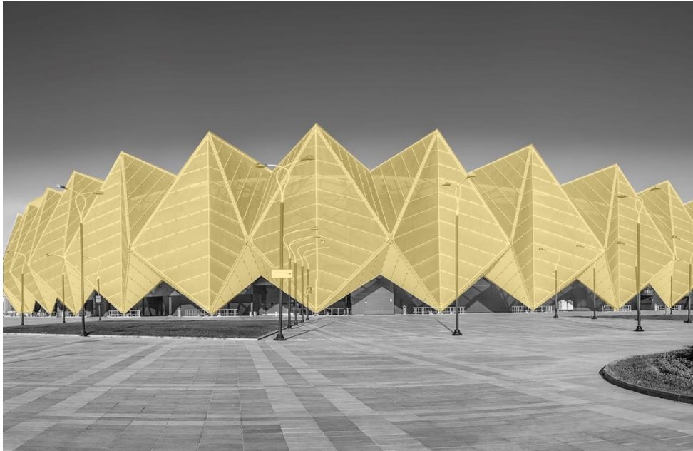
Figure 9. Structural and visual dynamism of Crystal Hall, Baku, 2013.
