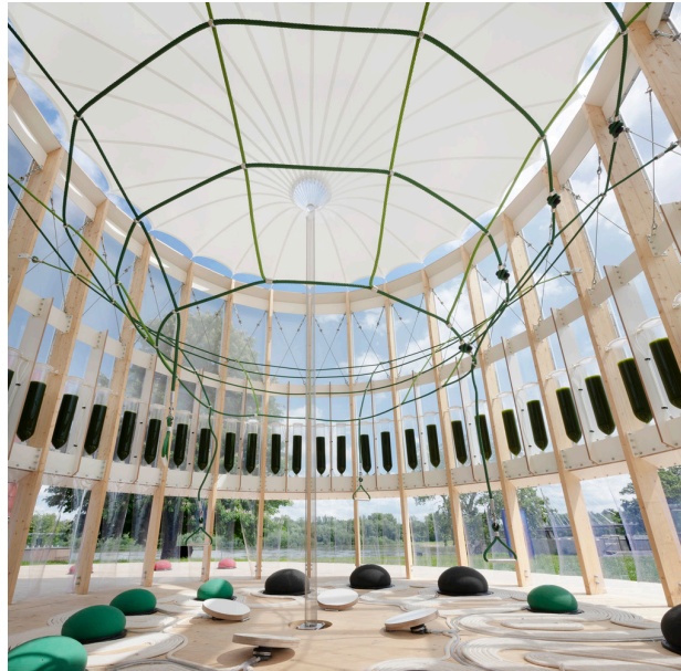
Figure 6. ecoLogicStudio, AirBubble , 2021, Bio- digital installation, Automated sensorial system, bioreactors, timber, ETFE membrane, Copernicus Science Center, Warsaw (Archdaily).
