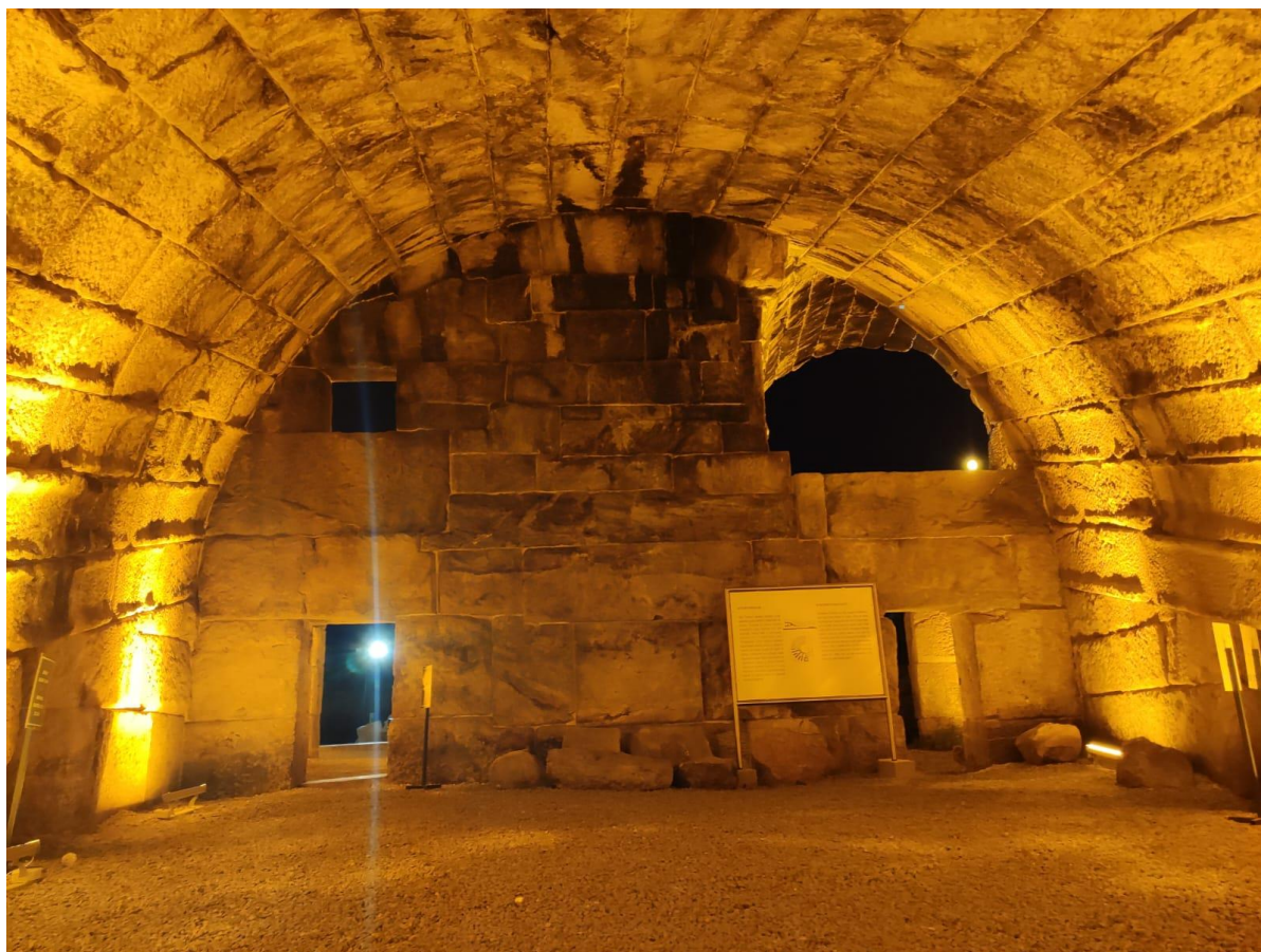
Fig. 6: Transitions from trapezoidal vaults to barrel vaults.
